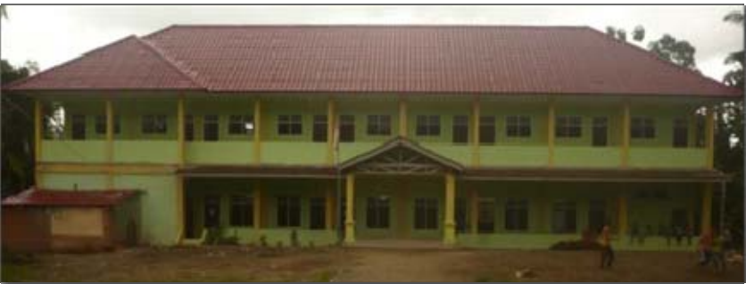
The completed Nias School Project Phase 1 and Phase 2
